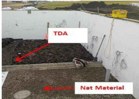
placing TDA in the southern half and natural material on the northern half of the ground
