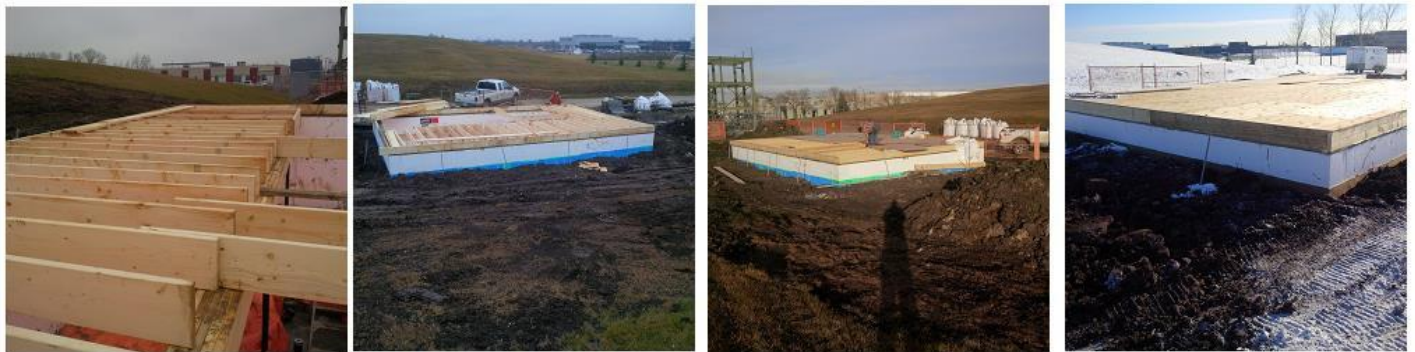
Framing of the floor joists
