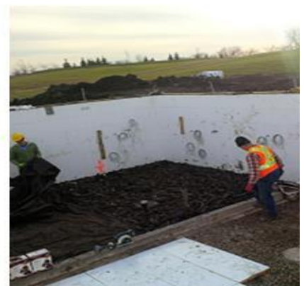
placing TDA in the southern half and natural material on the northern half of the ground
