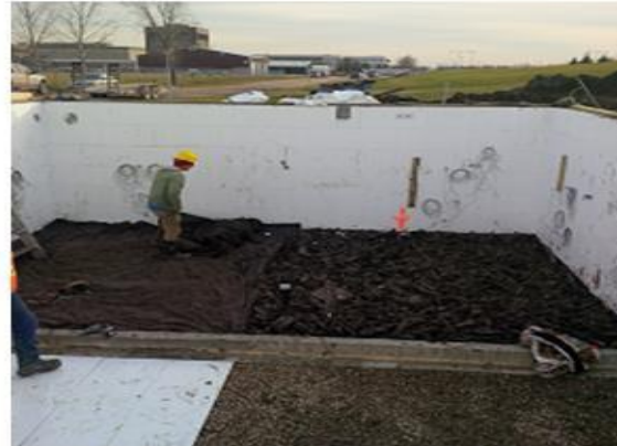
placing TDA in the southern half and natural material on the northern half of the ground
